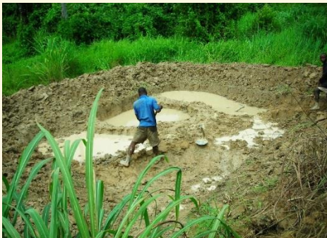
Manual construction of earthen pond
